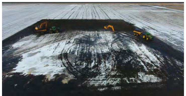
Figure 3. Farm Reservoir Installation
