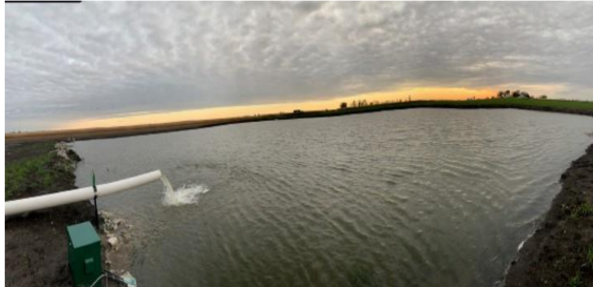
Figure 6. Completed Farm Reservoir
