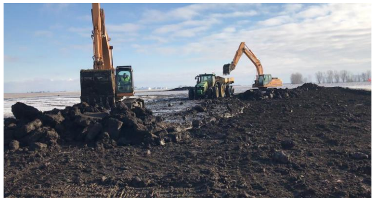
Figure 2. Digging of “Farm Reservoir”
