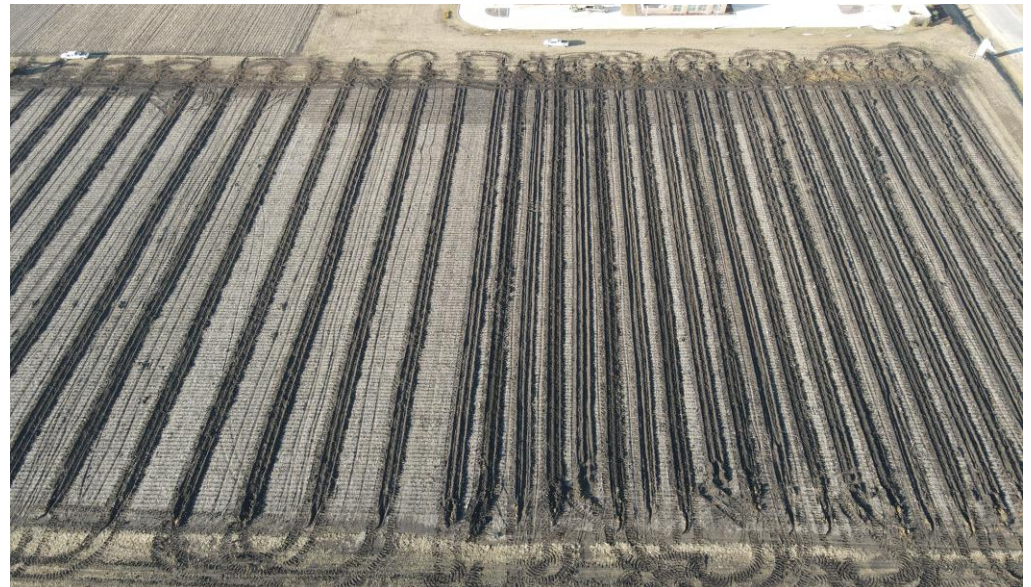
Figure 2. 15' and 30' Pattern Tile Installation
