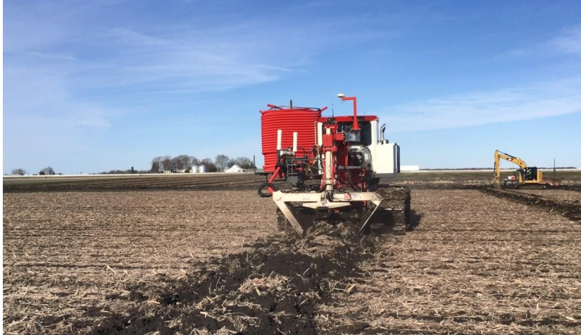
Figure 1. Tile Installation
