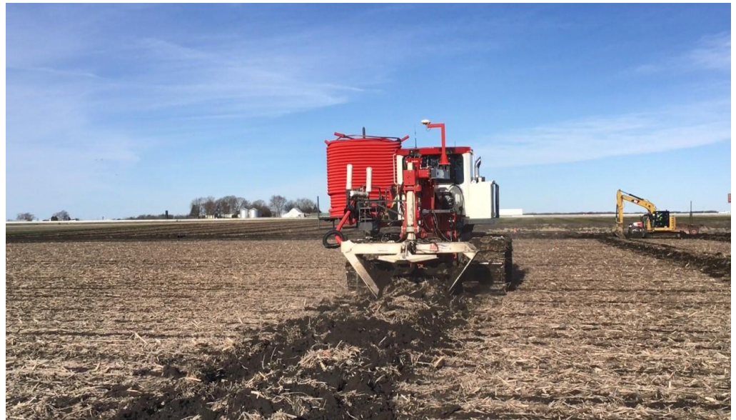
Figure 2. 15' and 30' Pattern Tile Installation
